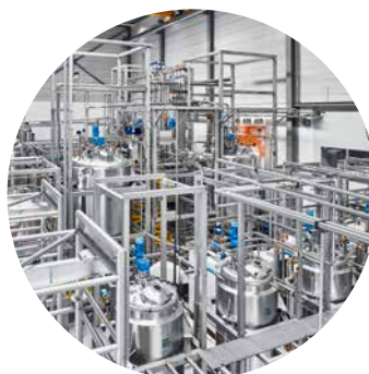
Modular Plant Construction
